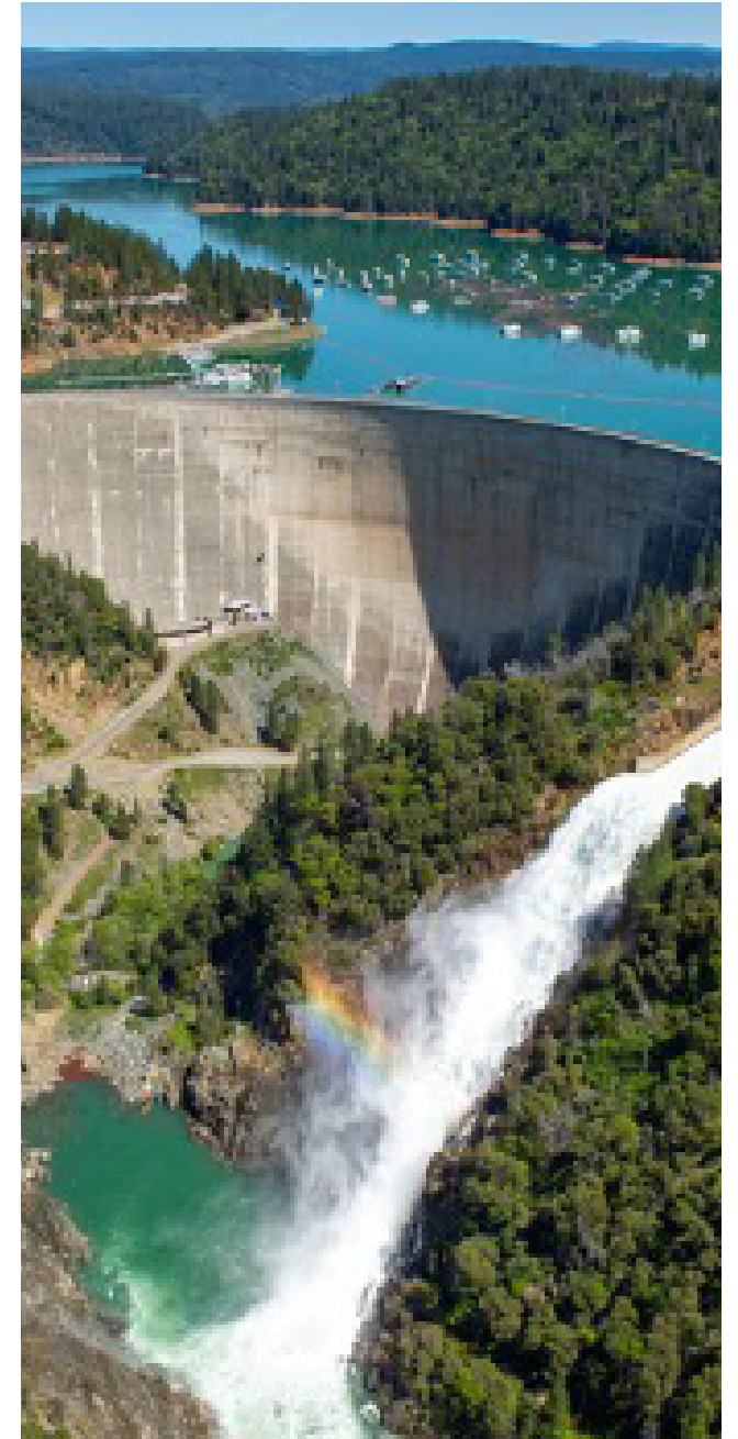
Image courtesy of Yuba Water Agency
